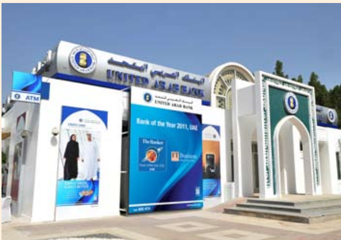
UAB's Ajman branch upon reopening after undergoing complete refurbishment.
